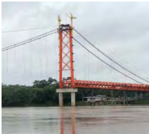
» Billinghurst Bridge, Peru
