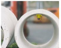
Drop pipe lifting sling through hole in pipe. Align and insert "Tea Cup" pipe carrier into lifting sling. Once set, you are ready to lift the pipe.
